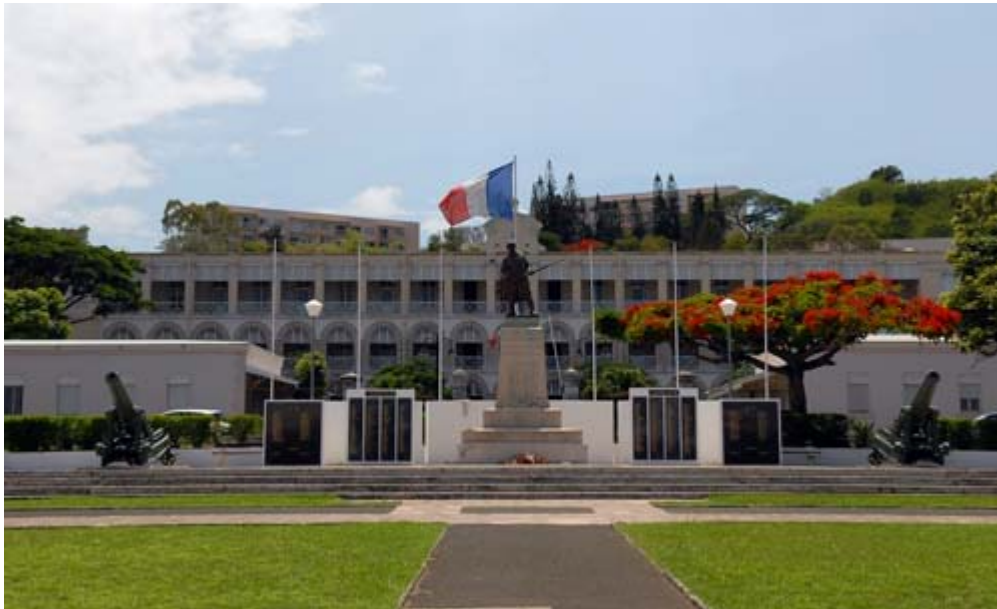
Shumeikan Headquarters - Noumea French Military Administration Bldg
